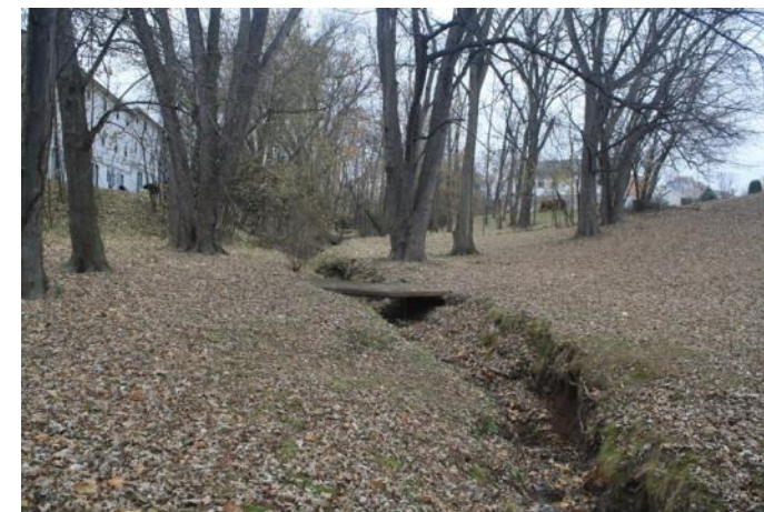
Photograph 4. Straightened, incised, and undercut streambanks with concrete slab bridge crossing, looking upstream.
