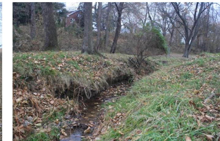
Photograph 5. Incised stream channel disconnected from a functional floodplain with 3.0' to 4.0' eroding and undercut streambanks with concrete slab encroachments in background, looking upstream.
