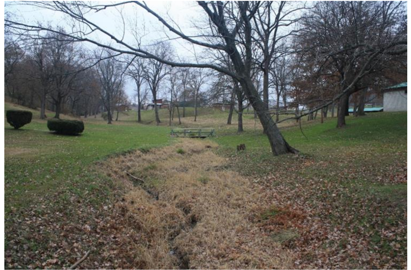
Photograph 7. Fairly well-connected stream condition near downstream wooden bridge, looking upstream.
