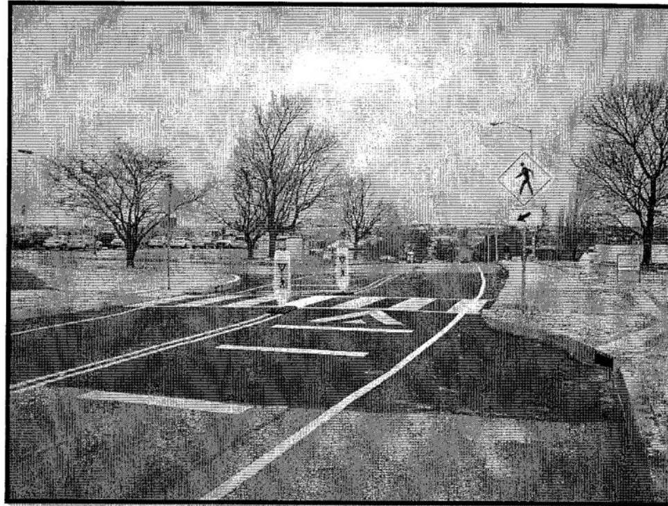
Figure 3: Example of a Raised Crosswalk in York, PA
